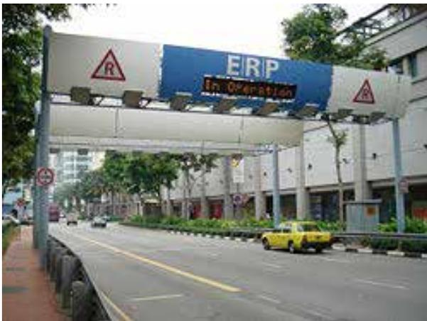
Different charges for different roads at different times are automatically deducted from the ERP "CashCard" as vehicle passes under gantries. The CashCard is fixed to the vehicle windscreen and can be bought/topped up at retail outlets, banks, petrol stations and automatic machines.
